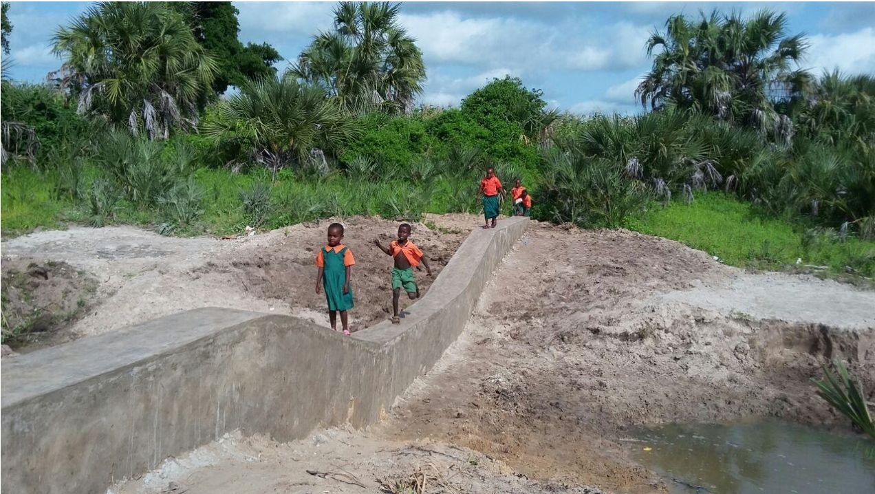
Bomani sand dam implemented by LKWRUA and WRA
