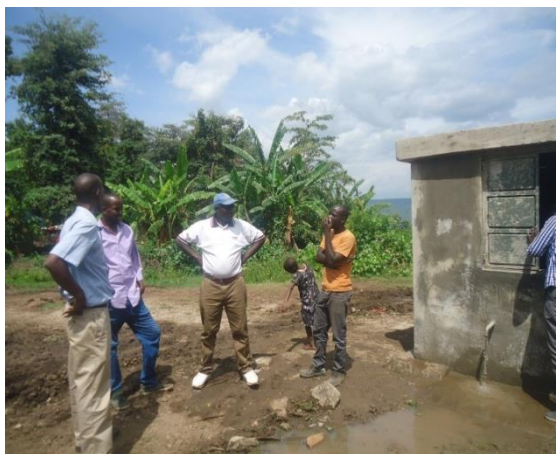
Asao WRUA conservation of springs with cattle trough and water kiosk in a well conserved catchment
