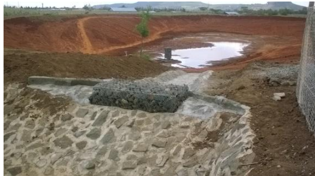
Gituamba dam: After rehabilitation
